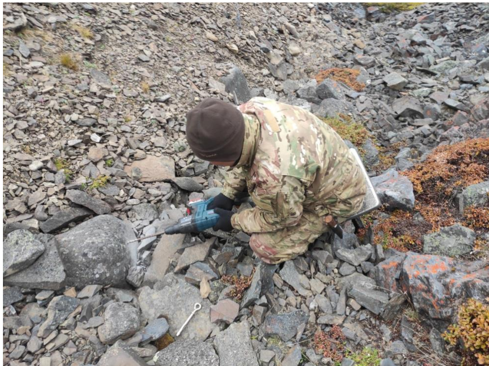
Fig.6. Fixing the trap to the stone with a perforator.
